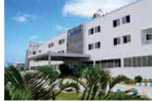
Rudrapur Plant (Green Building)
