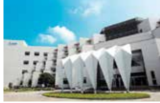
Tainan Plant (Diamond-rated Green Building)
