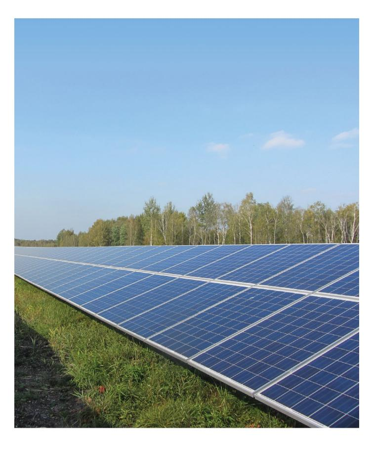
Reference installation in Lauchhammer (Germany): 3.83 MW nominal output power - 15,968 solar modules - 135 Delta string inverters
